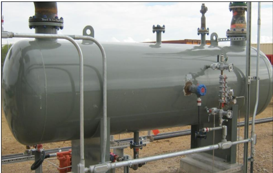
Figura N° 2.8 KNOCKOUT DRUM
