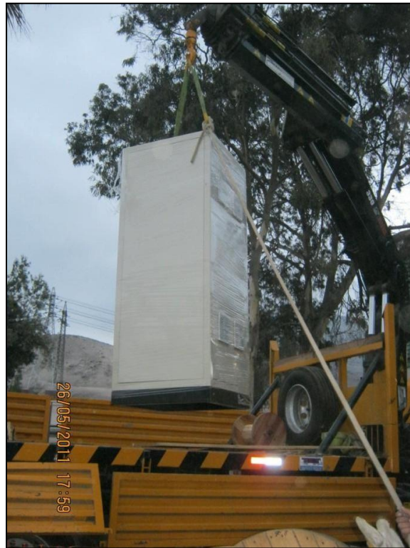
Fig.2.4: Montaje Tablero UPS
