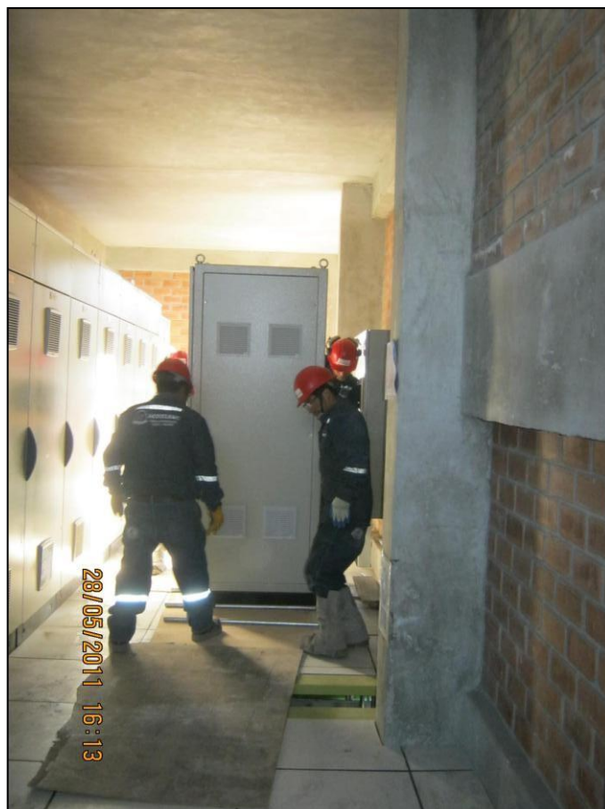
Fig.2.4: Montaje Tablero UPS
