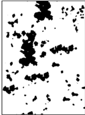
Rust Grade 3-G, 16% Rusted
