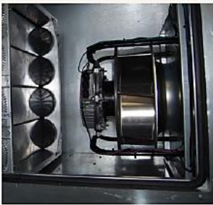
Electronically Commutated Motor (ECM) variable speed direct drive backward curved plenum fan ▼
