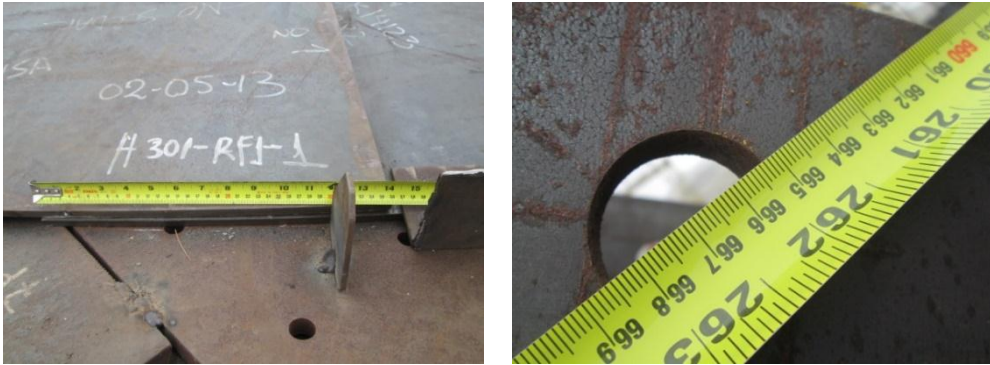
Control dimensional post soldeo /perforaciones
