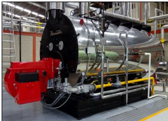
Figura 2: Caldera Piro tubular POWER MASTER
