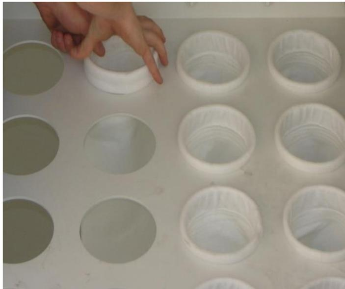
Figure 3. Typical bag installation.
