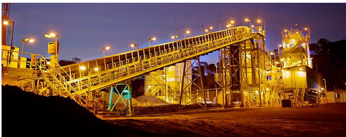
Figura 1-4: Zinc and Lead – Glencore
