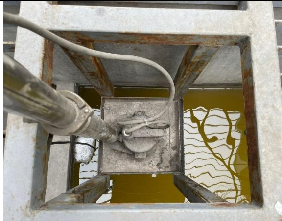
Foto 9: Electrobomba sumergible 2hP.
