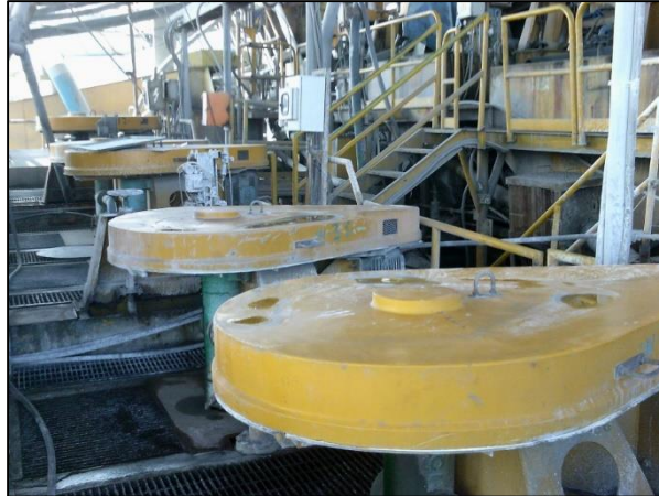
Figura 2.37 Celdas ok – 5 (scavenger) (C1)
