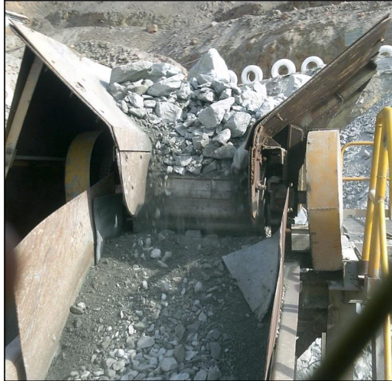
Figura 2.1 Apron feeder (AF)
