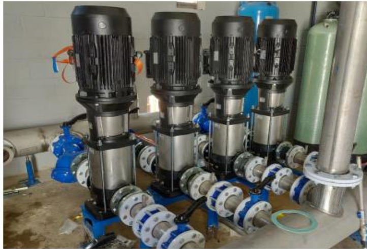
Figura 2-15 Bomba Centrifuga Vertical
